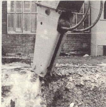
HM 305 "vibrosilenced" demolition of foundations
